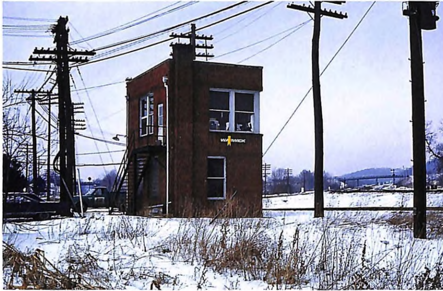
AT LEFT ABOVE: The yellow flag is displayed for a southbound train to pick up 19 orders at Warwick in February 1972. This picture gives a good overview of the track arrangement at Warwick. The Akron Secondary Track passes directly in front of the tower. South to Orrville is to the left. The B&O main line curves off to the right. B&O's CL&W Subdivision is visible along the pole line in the distance to the right of the tower. Richard E. Jacobs photo, David P. Oroszi collection
